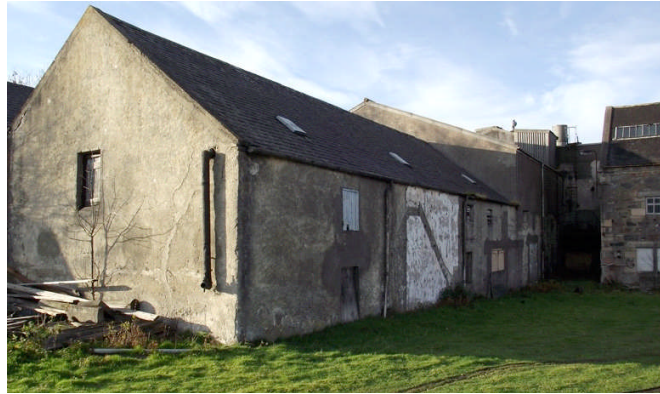
Fig. 7 : Malt barn and steeps buildings
