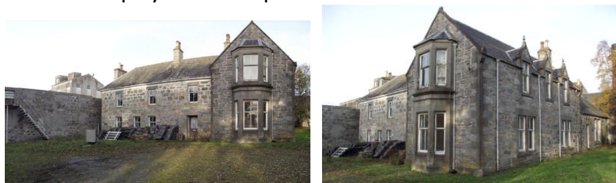
Figs. 5 and 6 : uninhabited residential property, which is proposed for demolition
